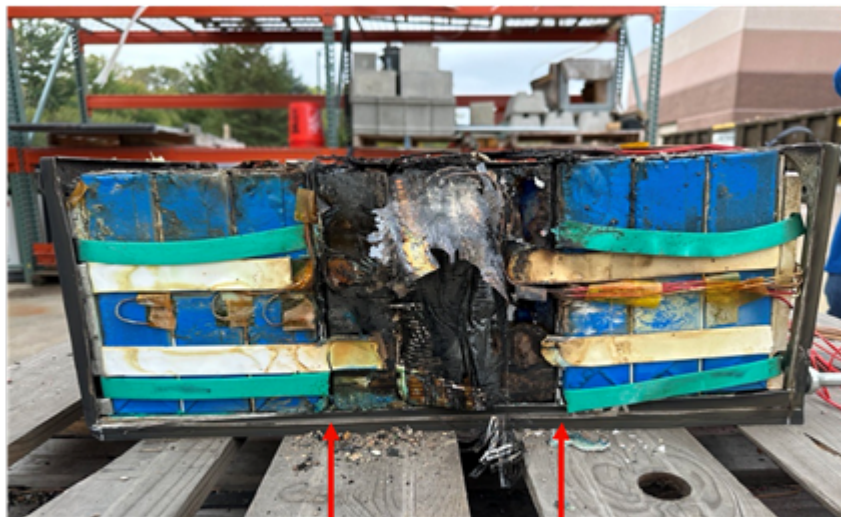
GORE Battery Insulation placement
